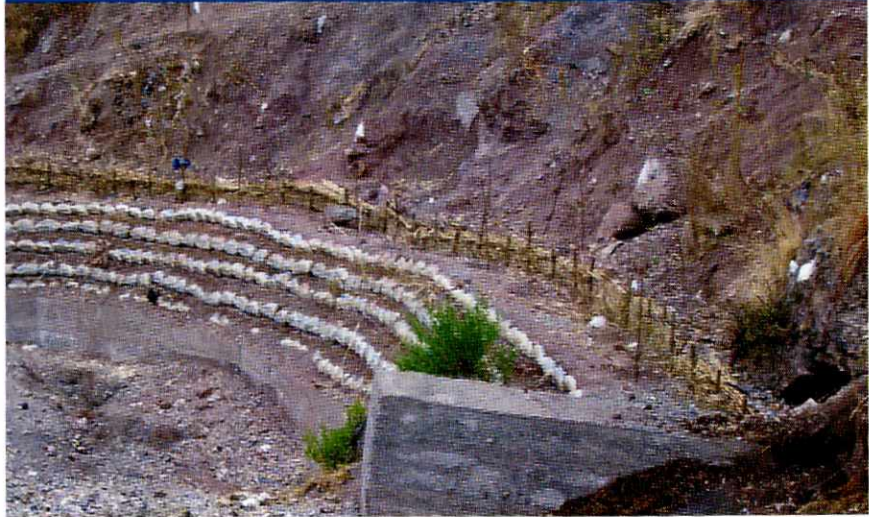
Combination of concrete, vegetated soft gabion and live brushwood R. Walls
